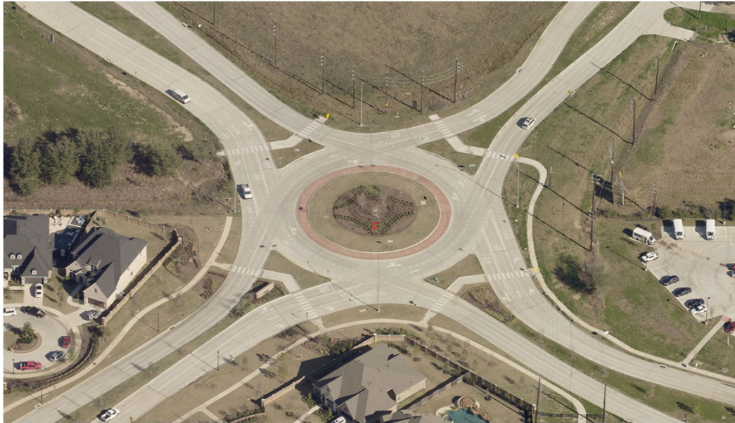
Upgraded 2-lane Concrete Roundabout with Storm Sewer
