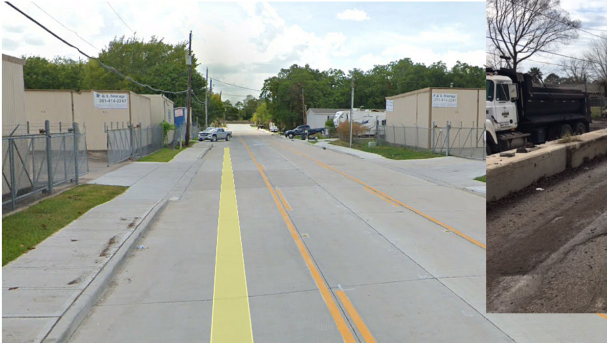
Upgraded 3-lane Concrete Roadway with Storm Sewer
